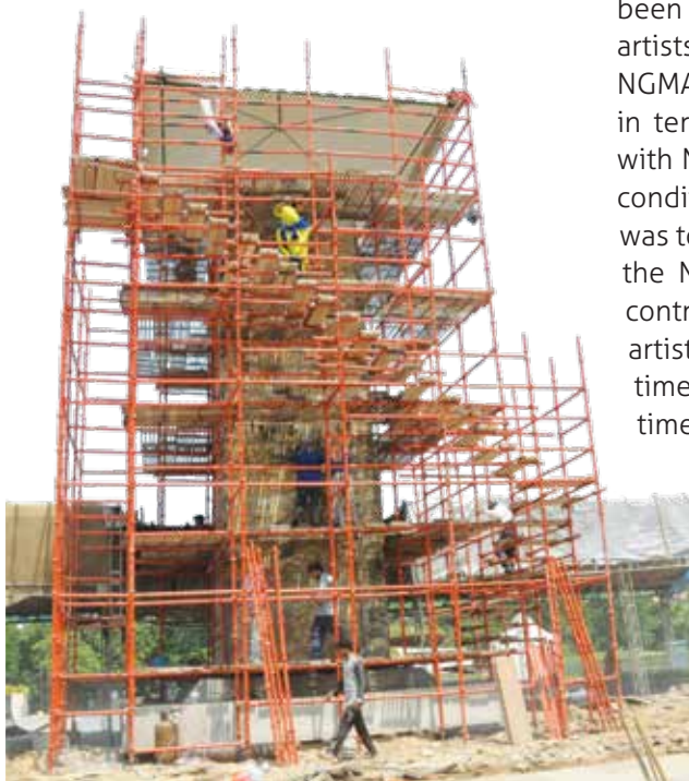
Scaffolding around the stone for NGMA artists to work.
