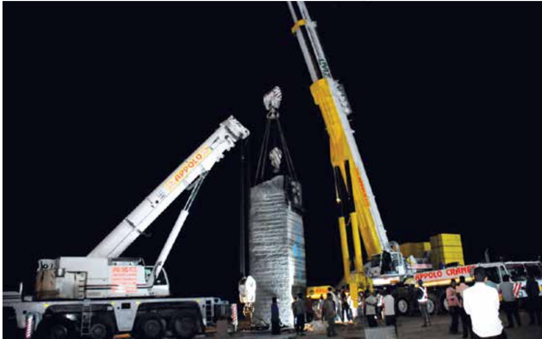
The 30 ft stone being lifted with two big cranes.
